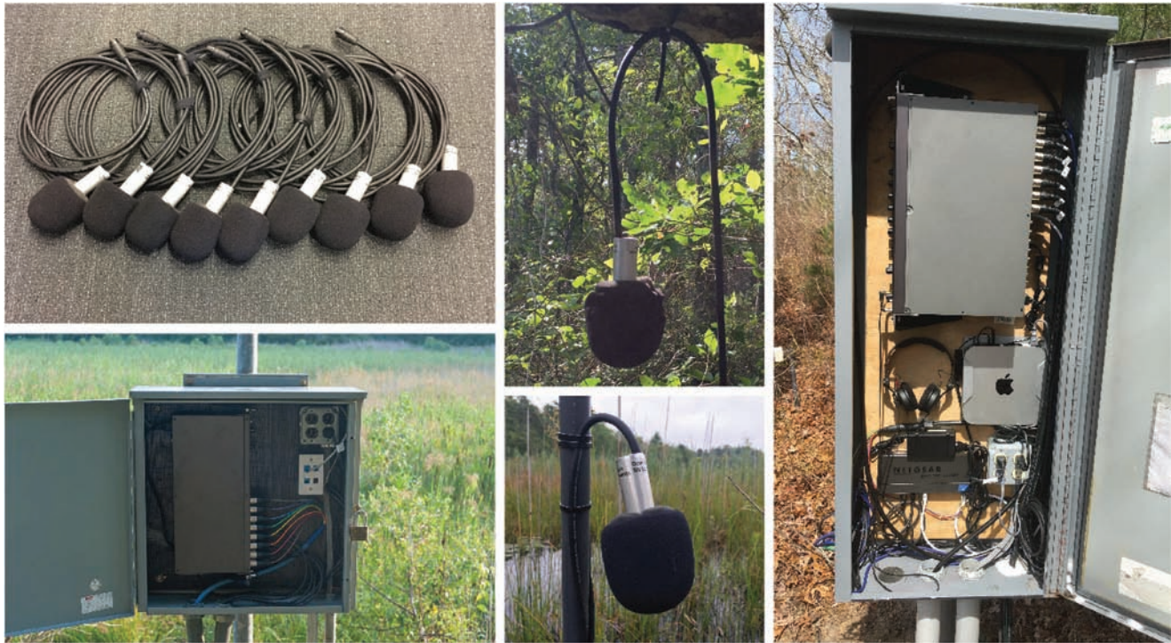
Figure 6. Parts of the audio streaming installation. Top left: microphones awaiting installation. Bottom left: satellite input box. Center: microphones in trees and in the marsh. Right: main electrical box, showing mixer (top), computer (center), network switch and fiber (bottom left).
